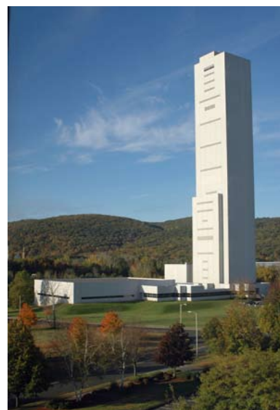
The Otis Elevator test tower in Bristol, CT is the tallest such tower in North America and could be seen from the convention hotel.
